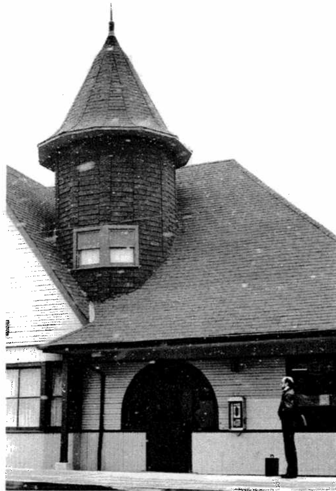
A 1889 drawing (left) of the 91st Street Station indicates the original Queen Anne-style details. Above, a contemporary photo of the station.
